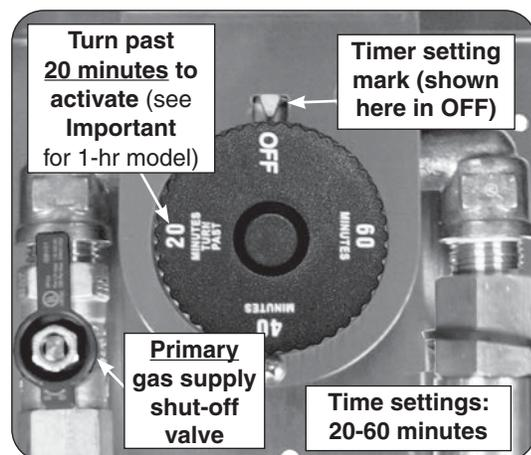
Fig. 3-1 1-hour timer operation
